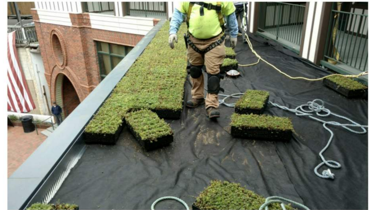
MODULAR PLANT TRAYS GREEN ROOF REFERENCE
